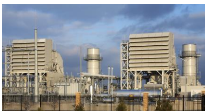
Invenergy's Cannon Falls Energy Center, located in Cannon Falls, Minnesota.
